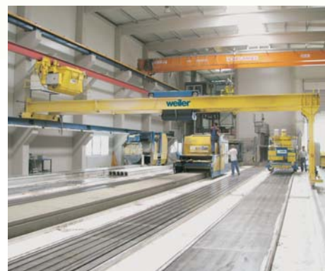
Automated concrete distributor
