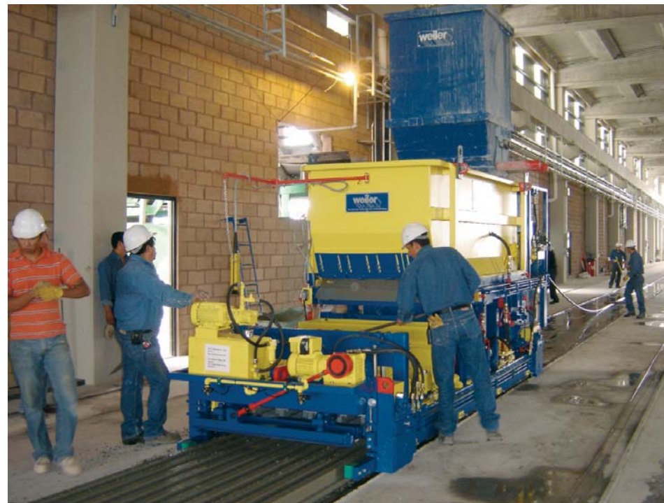
Placing of concrete
